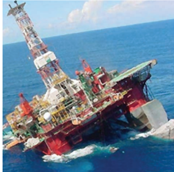
Offshore oil platform
